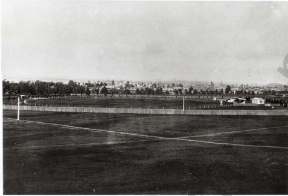
Figure Photograph by Captain Samuel Sweet, c.1877, depicting the Adelaide Oval with extant fencing and buildings, looking southwards towards Adelaide from Pennington Terrace with no vegetation in the foreground. Source: ACC archives; Mortlock Library B9138.
